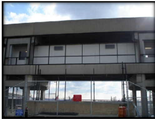
Figure 10: Temporary Connector Bridge
