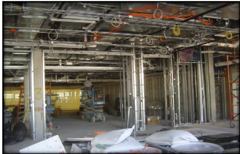
Figure 3: Ductwork obstruction in plenum space
