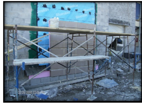
Figure 6: Cast stone mockup
